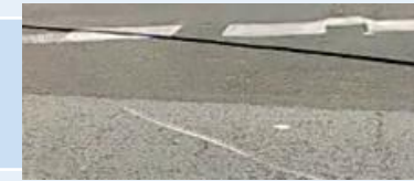
Transversal Construction Joint
