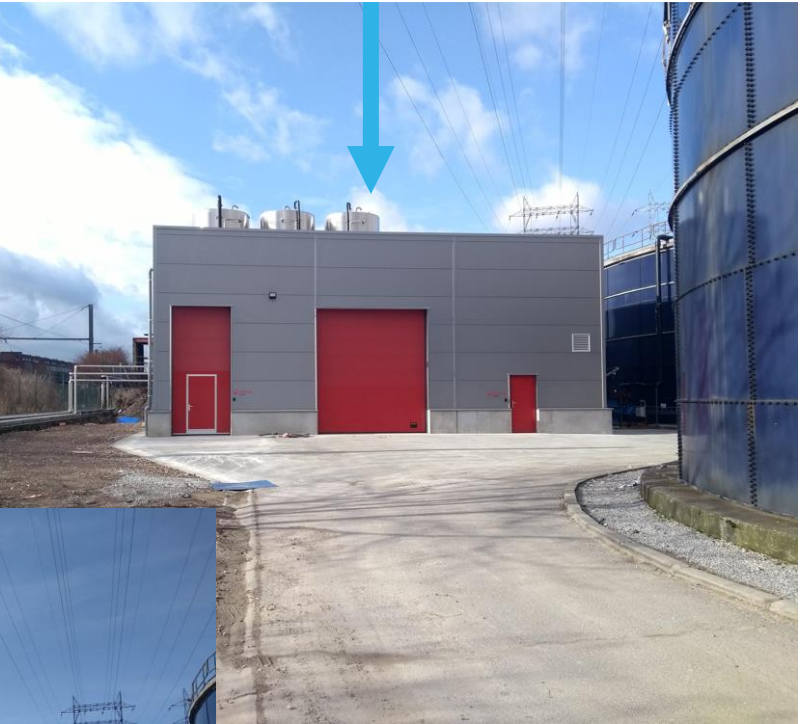
Water Reuse Building
