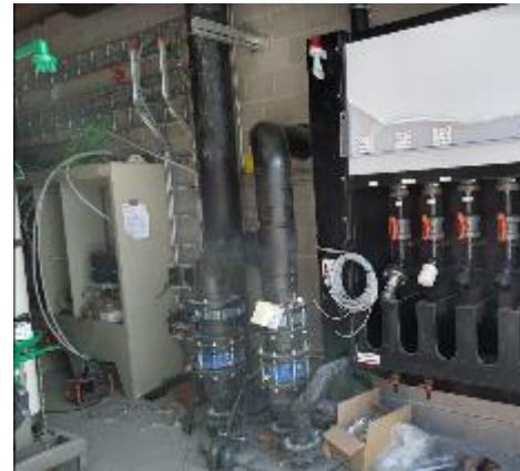
Hydraulic and electric assembly on site
